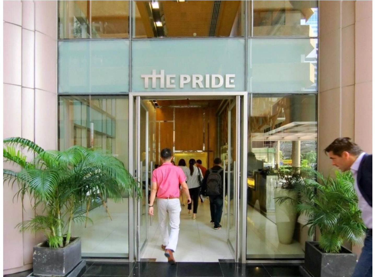
Office building main entrance
